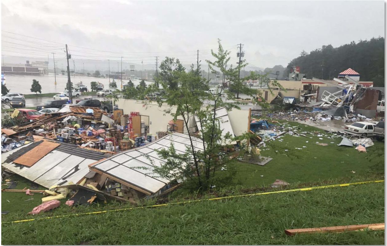
ABC Store #17 in Fairfield was destroyed by a tornado on June 22, 2017.
